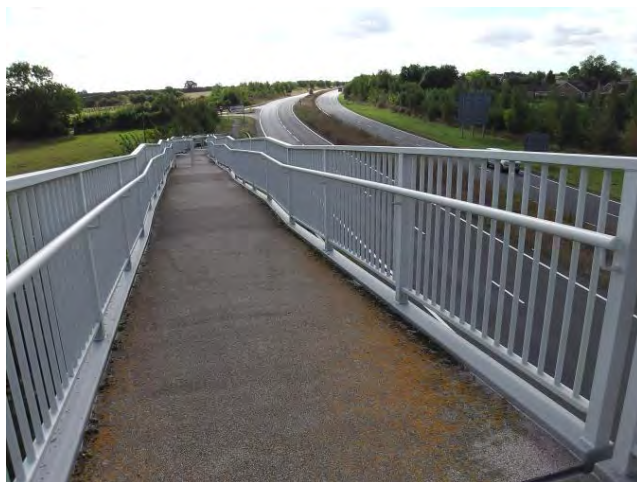
Footbridge across A6 at Stanwick Road
